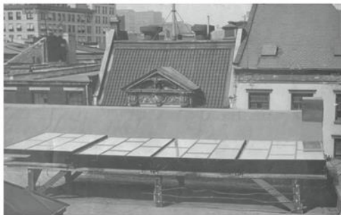
Figure 21.6. Charles Fritts put up the first photovoltaic array, in New York City in 1884.
